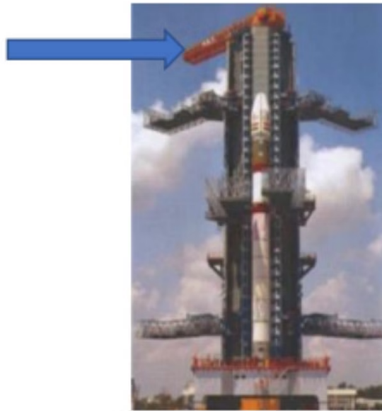
10 T Hammer Head Tower Crane
